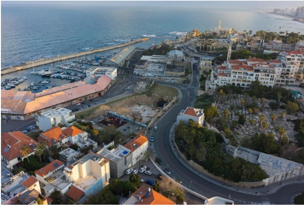
Figure 9. The Jaffa hill from the south. To the left, the 'Ajami neighborhood that began as one of the Egyptian settlements on Jaffa's immediate periphery. To the right, the old Jewish cemetery. Photograph by the Griffin Company, courtesy of the Israel Antiquities Authority.
